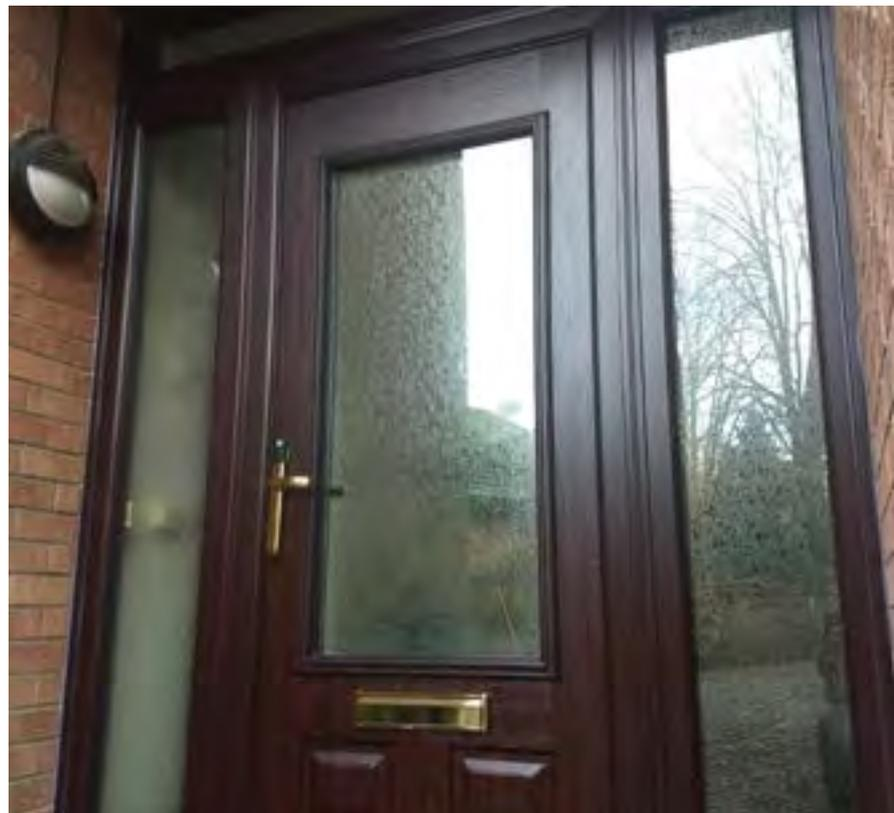
\*These are triple glazed and the patterned glass is an integral part of the design. It is encapsulated in the clear sealed unit and an alternative backing glass cannot be chosen.
