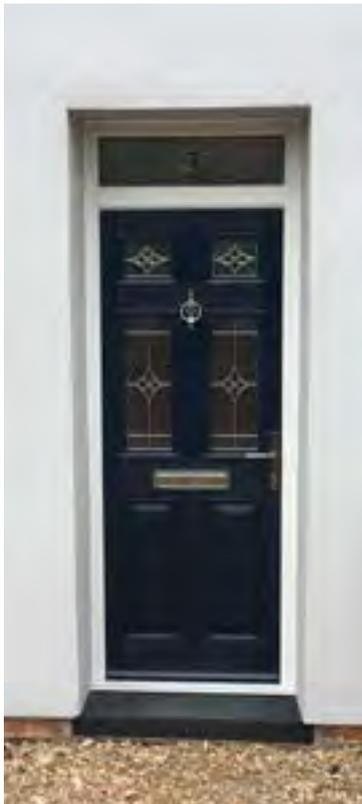
\*These are triple glazed and the patterned glass is an integral part of the design. It is encapsulated in the clear sealed unit and an alternative backing glass cannot be chosen.
