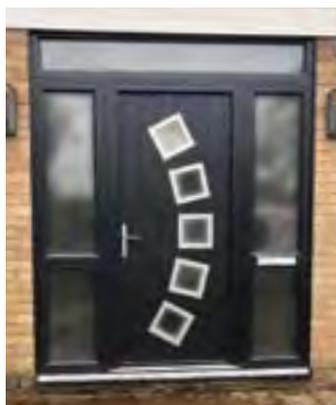
\*These are triple glazed and the patterned glass is an integral part of the design. It is encapsulated in the clear sealed unit and an alternative backing glass cannot be chosen.
